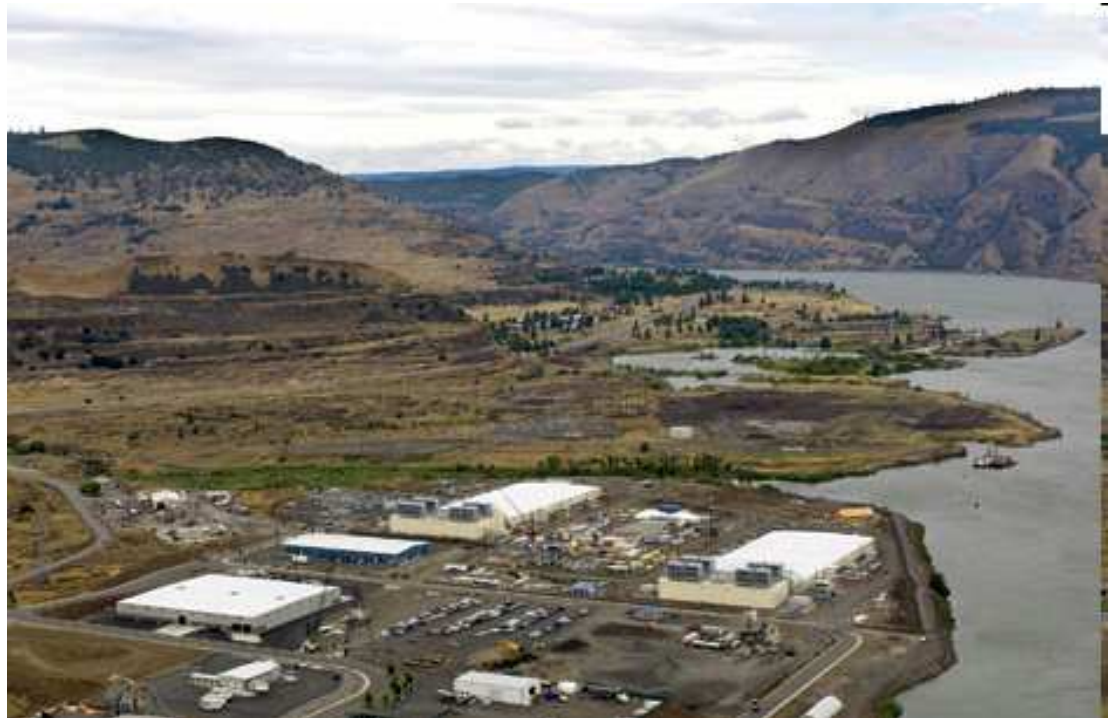
Google data center in Oregon
