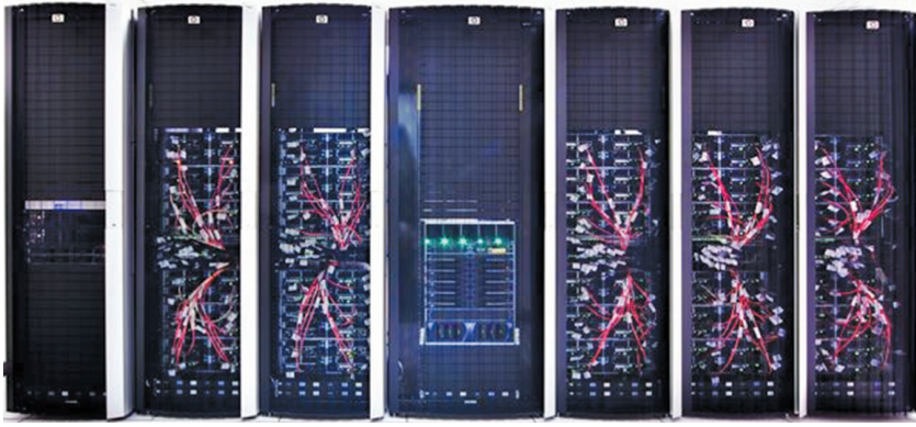
Figure 2. The KID system as installed in Keeneland's data center. The compact 201 teraflops/s system requires only seven racks and 90 square feet of floor space.
